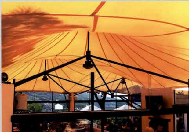
Natural translucency of the membranes blocks the UV but allows for natural light
